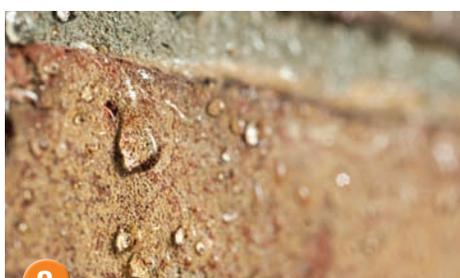
8 As Stormdry is formulated to penetrate deeply into masonry it can take up to two months after application for a noticeable “beading effect” to appear when rainfall strikes the wall. The masonry will be resistant to light rain after two to four hours.
