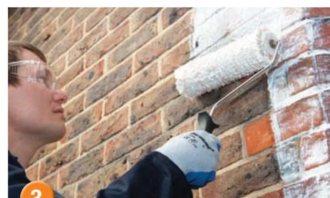
3 Larger areas can be covered more quickly using roller application. Stormdry can also be applied by electric roller or airless spray – call our technical department for details.
