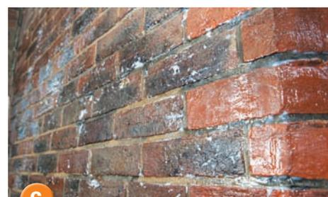
6 15-20 minutes after application, Stormdry starts to penetrate into the masonry and the whiteness will fade.
