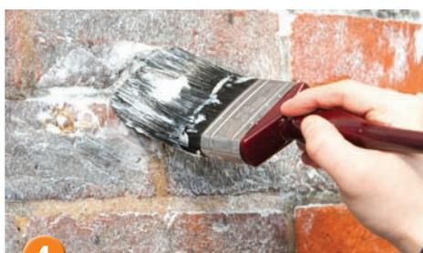
4 Check for any “missed” areas that have not been treated (e.g. voids in brickwork, deep mortar beds) and apply Stormdry to these areas using a brush.
