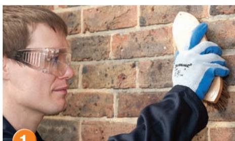
1 Carry out surface preparation as described in Preparation section. Remove any loose mortar, dust etc... using a masonry brush. When biological growth such as moss, algae or lichen needs to be removed, apply Soluguard Multi-Surface Biocide in accordance with instructions.
