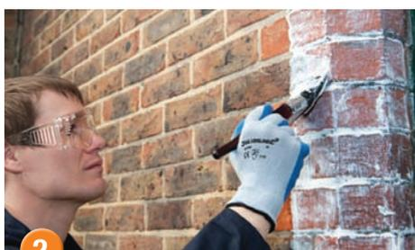
2 Stormdry can be applied by brush around details such as windows. Care should be taken to ensure that Stormdry does not splash onto glass, paintwork, plants, etc. Any splashes should be cleaned away with warm soapy water.
